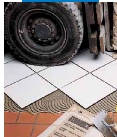
Rapid overlaying on asphalt industrial floor
