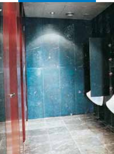
An example of an installation of marble walls with Keraquick - Feuchtwangen casinò bathroom (Germany)
