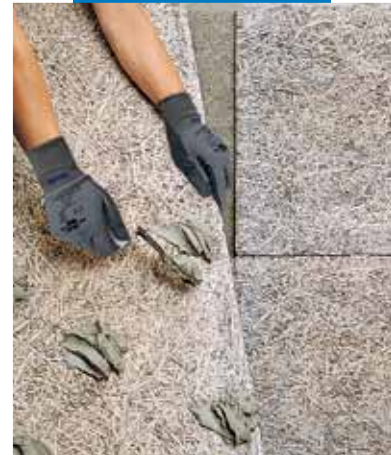
Laying heavy insulation panels
